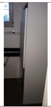
DHW tank deformation causing deformation of outer casing
